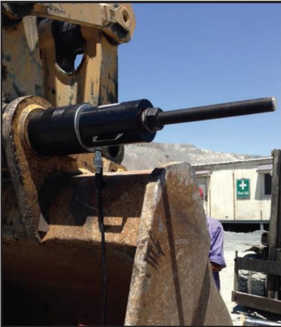
HPR-2 50 tonne kit in use on link pin removal.
